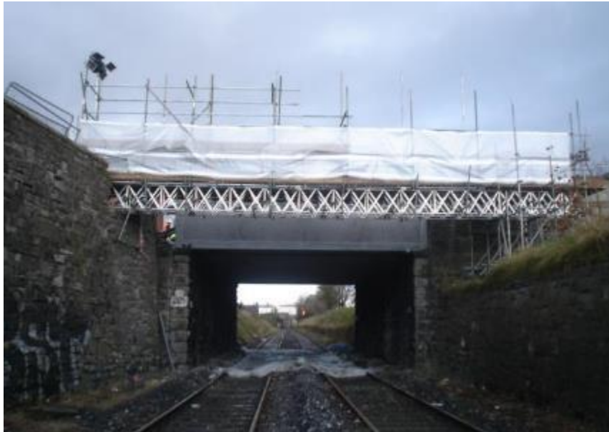
Figure 3-14 Scaffold for temporary diversion
