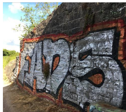
Figure 21 – North East wing wall.
