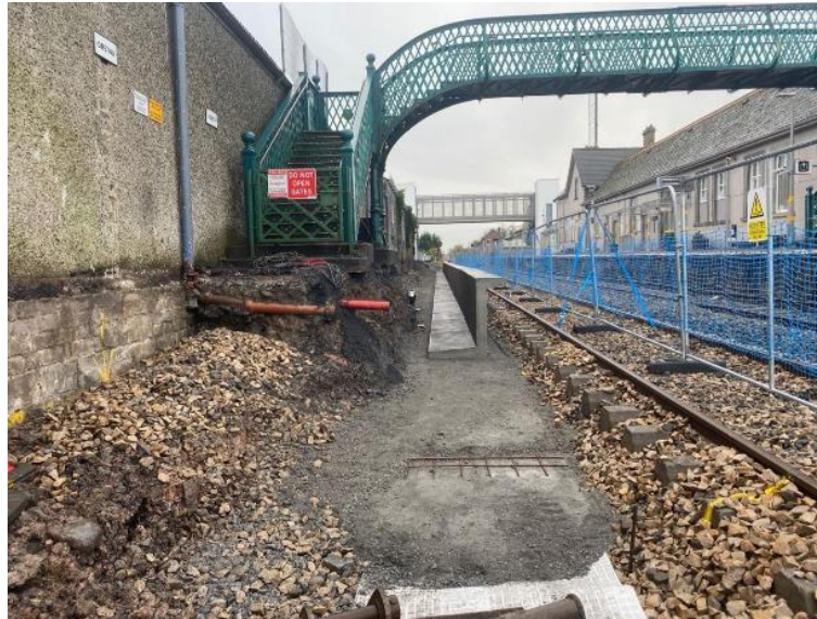
Figure 4-3 Example of track closure required to complete platform works
