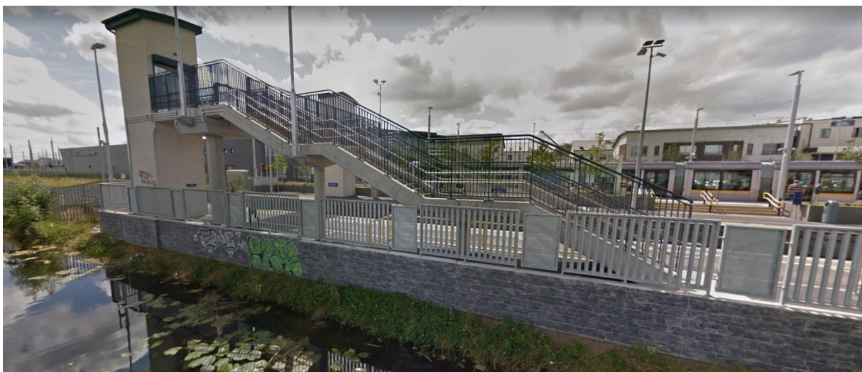
Figure 3-6 Existing footbridge OBG4A
