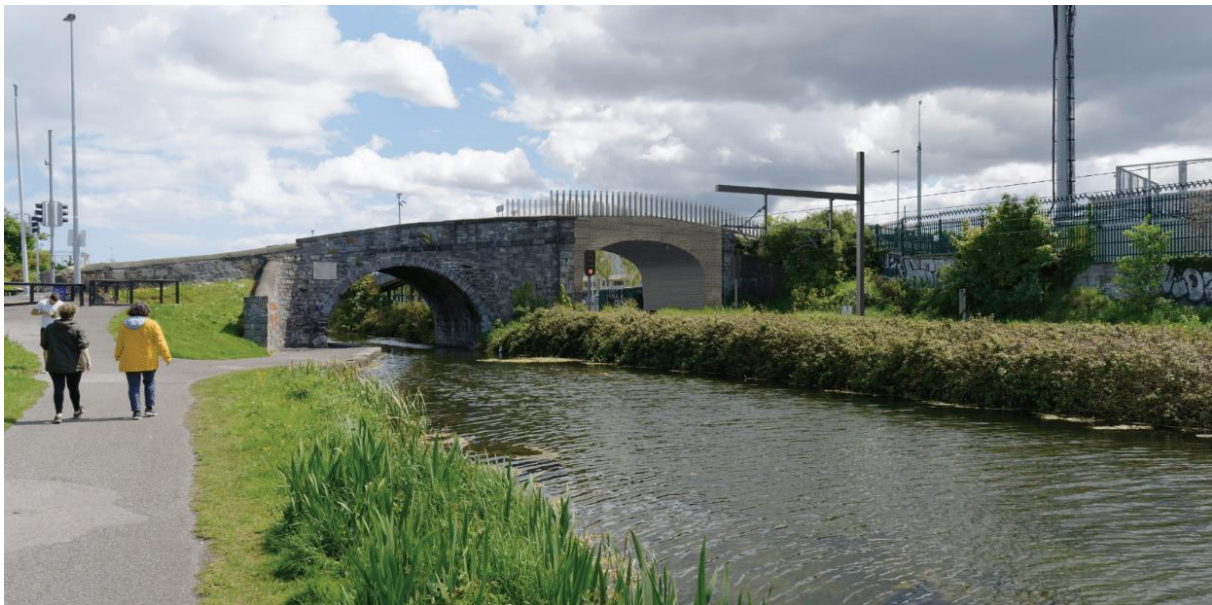
Figure 3-11 OBG5 Broome Bridge Photomontage - Canal View West
