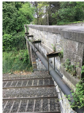
Figure 2 – East elevation of Castleknock Bridge, access restricted.
