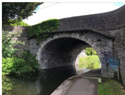
Figure 11 –Granard Bridge west elevation.
