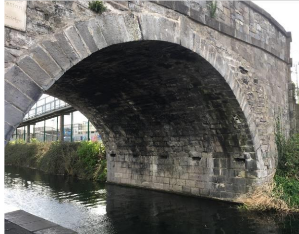
Figure 3 – West spandrel of bridge and canal arch.
