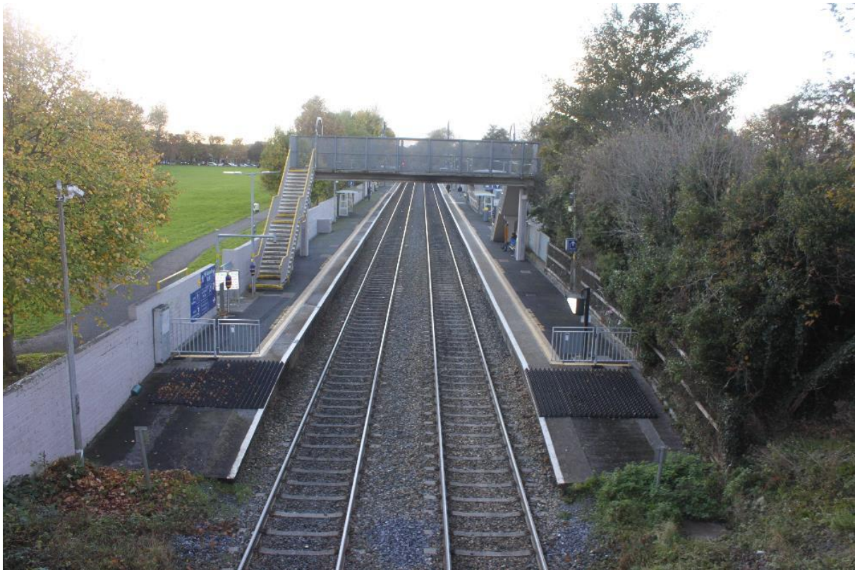
Figure 3-1 Castleknock platform view from OBG11
