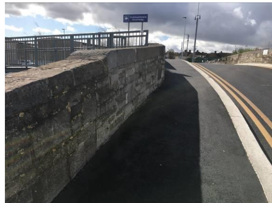
Figure 11 –View looking south over the bridge, with historic coping stones on the parapet.
