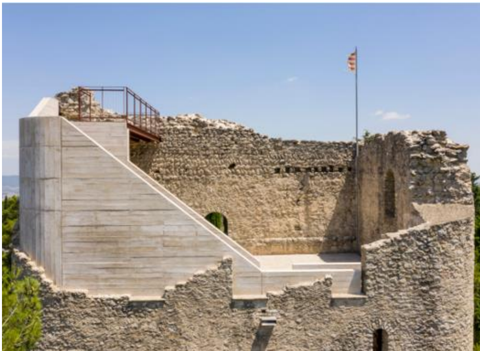
Figure 29 - Example of a new board marked concrete insertion in an existing stone structure.
