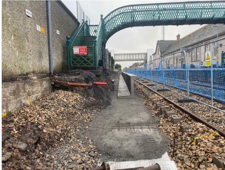
Figure 4-2 Example of track closure required to complete platform works
