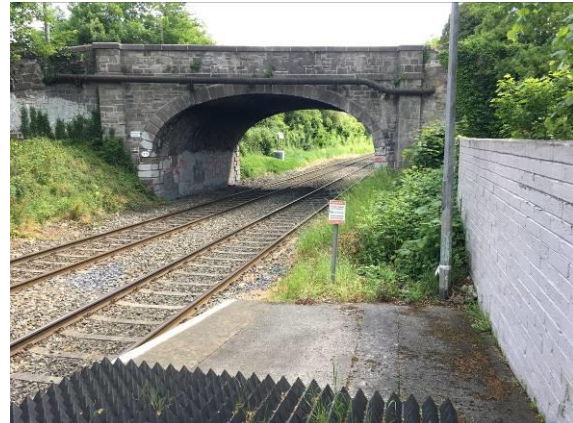
Figure 15 – West elevation of bridge.
