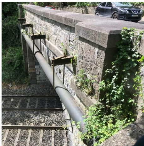
Figure 20 – East parapet with steel beams built in to historic stonework.
