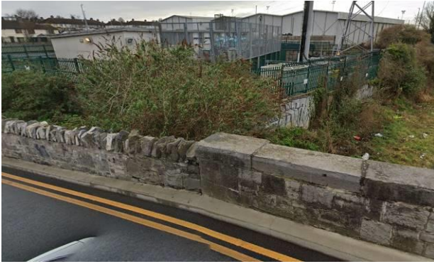
Figure 8 – South west parapet end and recently reconstructed random rubble limestone wall.
