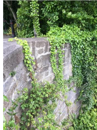
Figure 19 – North east wing wall parapet rebuilt in blockwork internally.
