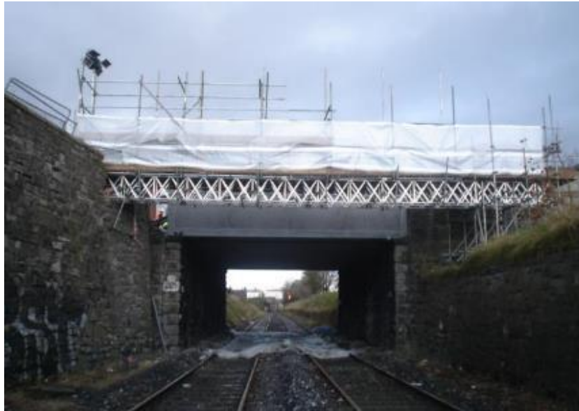
Figure 3-13 Scaffold for temporary diversion
