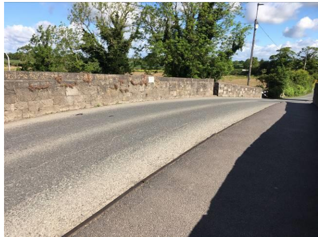
Figure 13 – View taken standing on crown of the bridge over the railway arch, looking north. Parapet over canal arch visible with gap between parapet and separate wall, in background.
