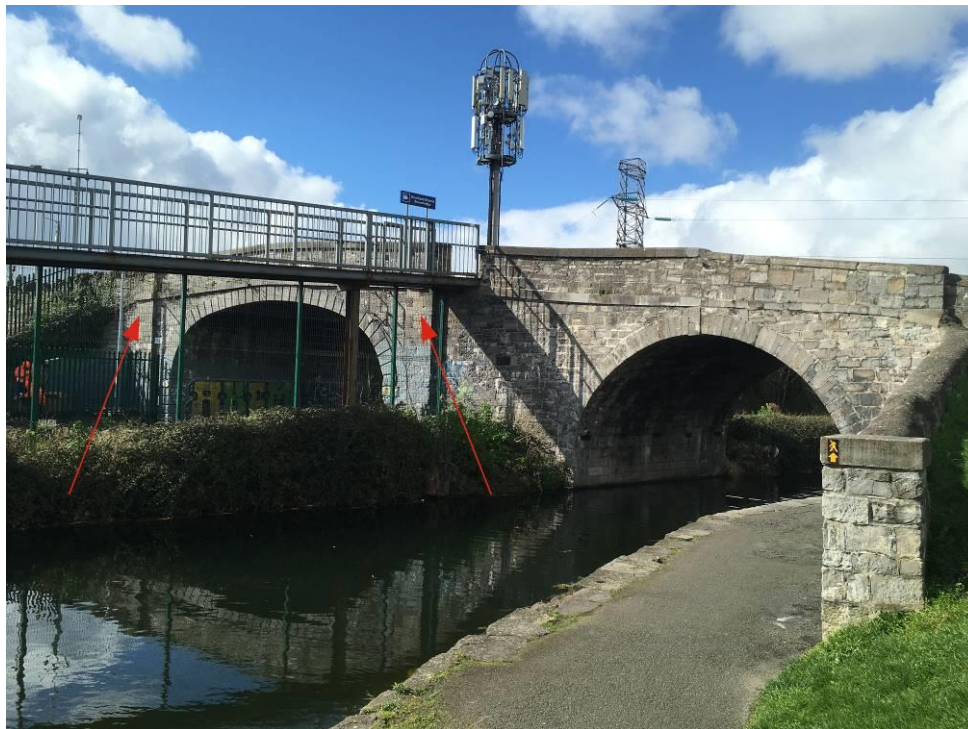
Figure 27 – Existing bridge with engaged piers highlighted.
