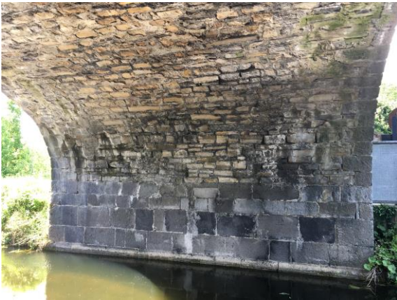
Figure 18 – Condition of arch stonework.
