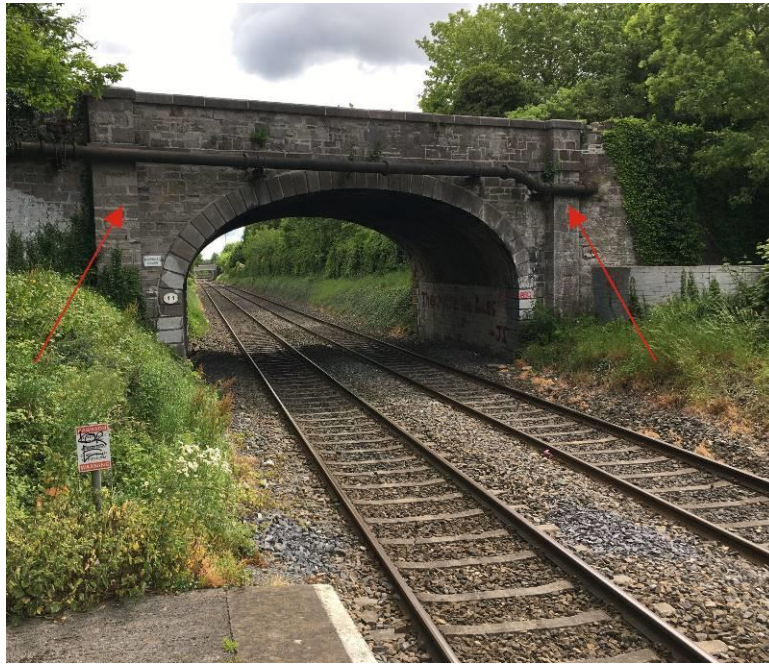
Figure 27 - East elevation with piers highlighted.
