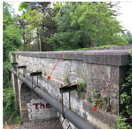
Figure 25 – East Elevation with string course highlighted.
