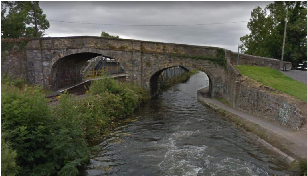
Figure 3-16 OBG 14 Cope Bridge view from the Royal Canal
