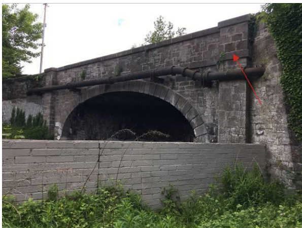
Figure 24 – West elevation with string course highlighted.
