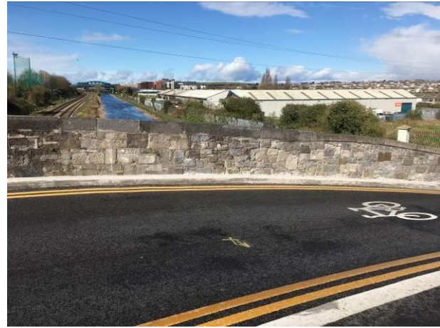
Figure 14 – West parapet showing section of parapet rebuilt.
