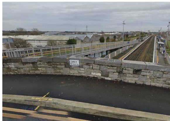
Figure 12 – East parapet and crown of bridge over railway line.
