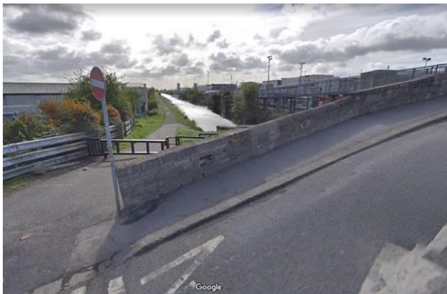
Figure 6 – North east wall, showing reconstructed end and path to the canal on the left side.
