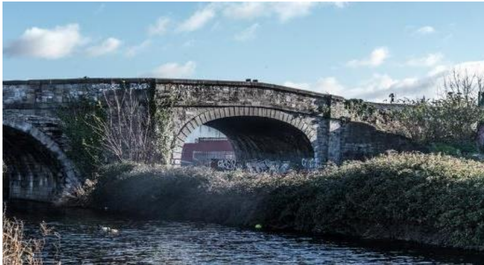
Figure 2-1 OBG5 – Broome Bridge
