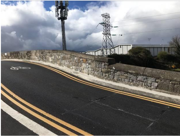
Figure 13 – Oblique view of west parapet looking south showing step where the parapet meets the adjoining wall and differing stonework styles and copings.
