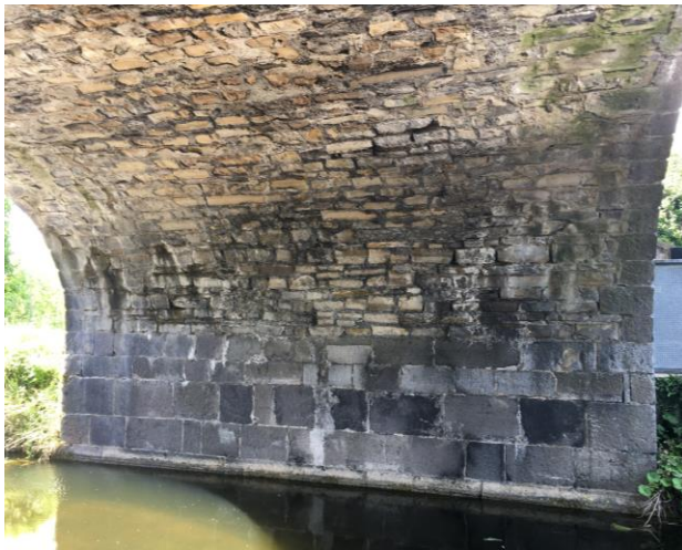
Figure 7 – Canal arch vault and south facing abutment of limestone ashlar.
