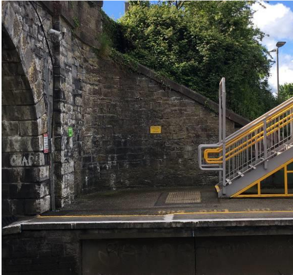
Figure 22 – South East wing wall.
