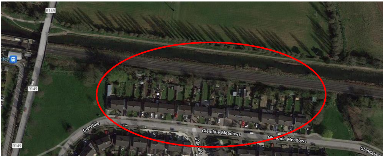
Figure 3-20 Houses affected by drainage works
