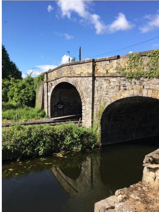
Figure 6 – Oblique view of east elevation.
