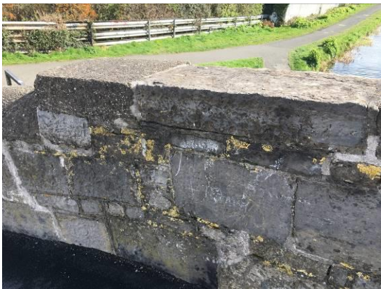
Figure 10 – East parapet wall over canal with historic limestone copings.
