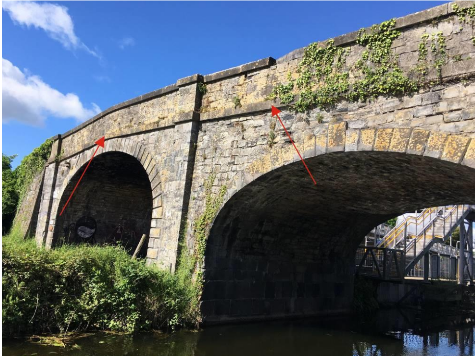
Figure 28 – Existing bridge with continuous string course over both arches highlighted.
