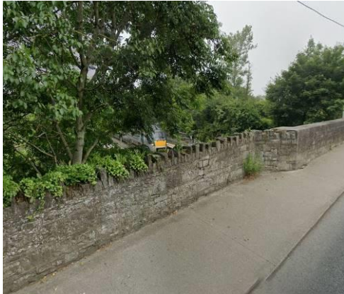
Figure 3 – West parapet ending with pier and historic boundary wall abutting.
