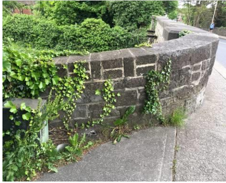
Figure 7 – North east parapet with modern blockwork.
