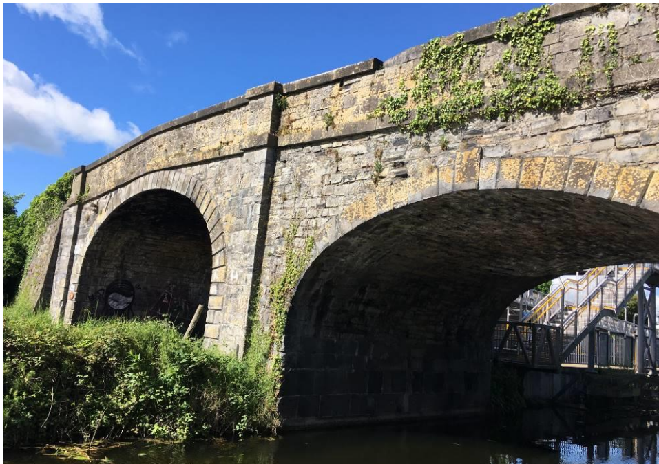
Figure 11 – Random squared limestone parapet and stringcourse across full length of bridge.
