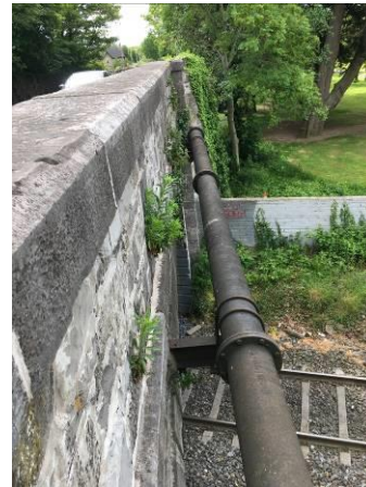
Figure 10 –West spandrel of bridge and canal arch.
