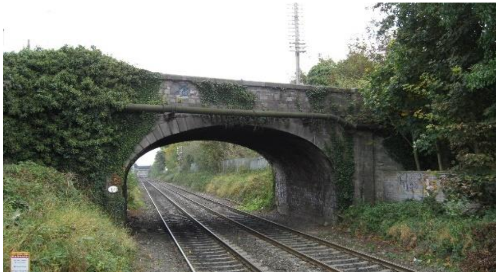
Figure 2-2 OBG11 bridge next to Castleknock Station
