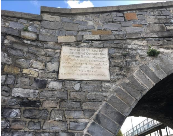
Figure 2 – Canal spandrel with squared limestone and commemorative plaque for Sir Hamilton.
