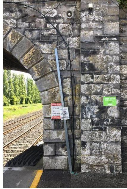
Figure 10 – West facing spandrel of the railway arch showing random squared limestone.
