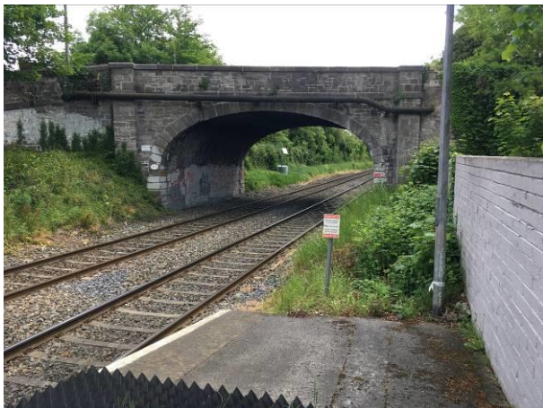
Figure 1 – West elevation of Castleknock Bridge over the railway line.
