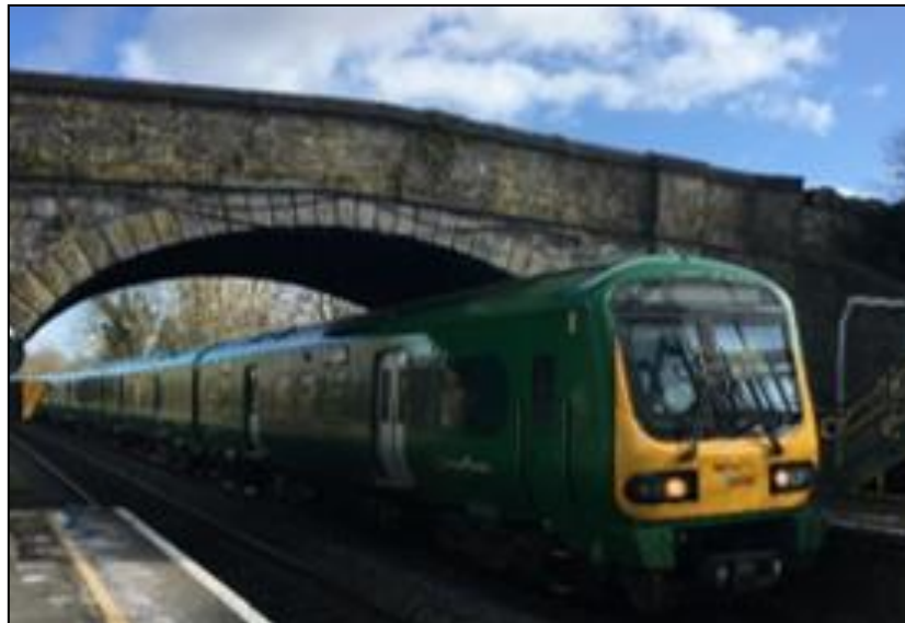
Figure 2-2 OBG14 – Cope Bridge
