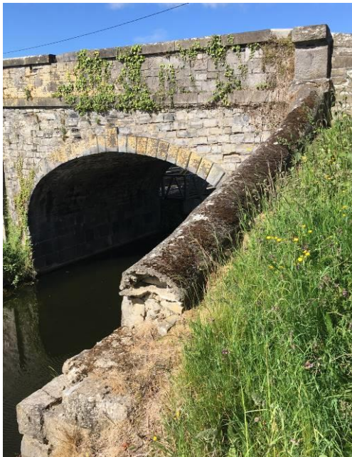
Figure 4 – North east wing wall with concrete flaunching.
