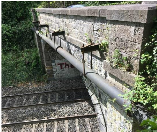
Figure 9 – Canal spandrel with squared limestone.
