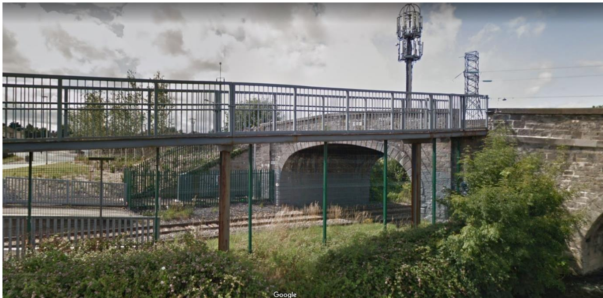
Figure 3-4 Existing access ramp to OBG5
