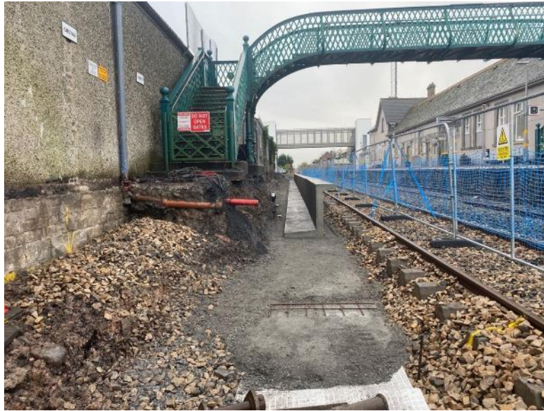
Figure 4-1 Example of track closure required to complete platform works
