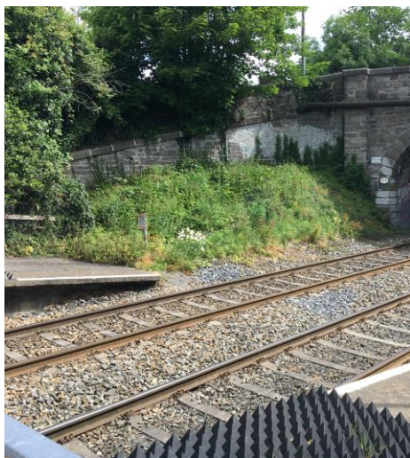
Figure 5 – North west wing wall.
