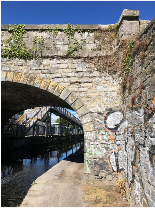
Figure 2 – East elevation showing arch ring.
