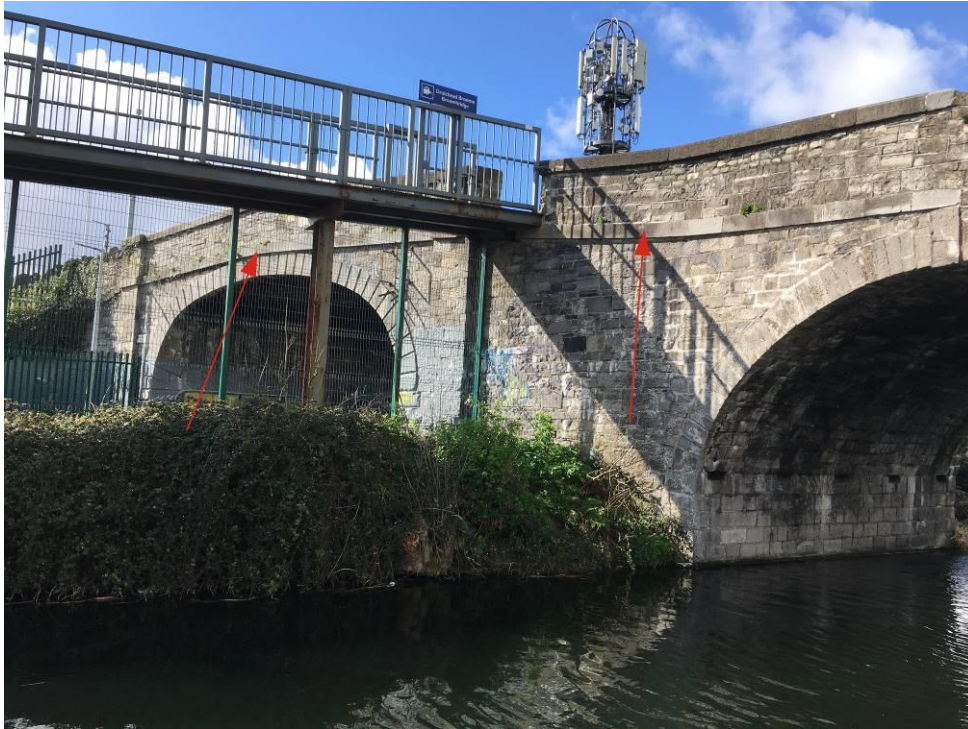
Figure 25 - Image of existing spans with string course highlighted.
