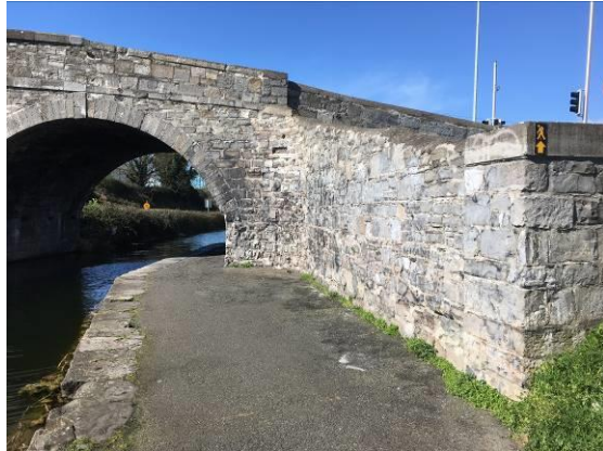
Figure 21 – North east wing wall.
